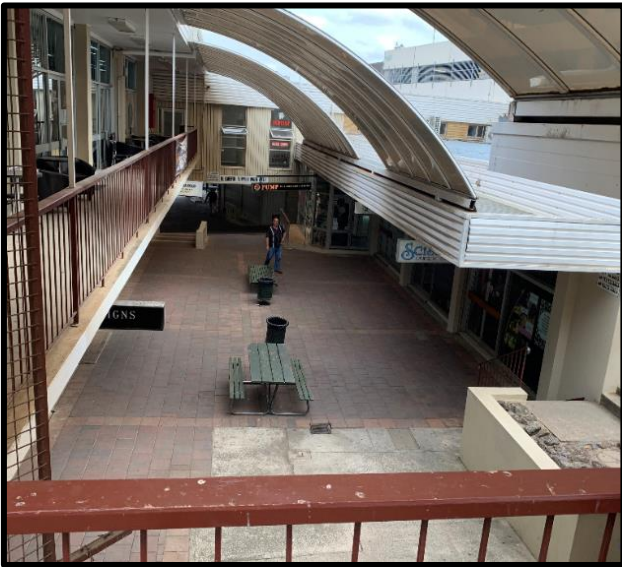
Image 10: Photo taken from the top floor. The site has an open ceiling.
