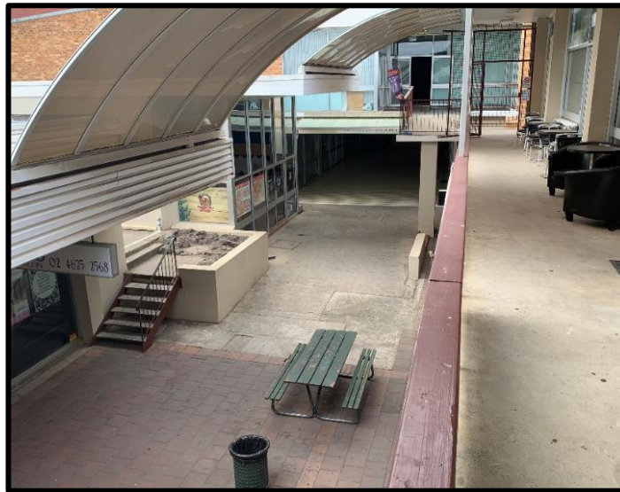
Image 11: Photo taken from the top level on site.
