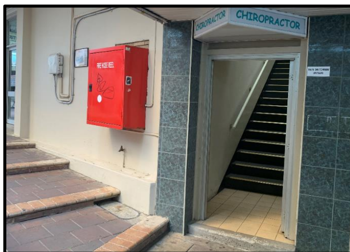
Image 5: One of the outlets within the site, located on the westside of the site.
